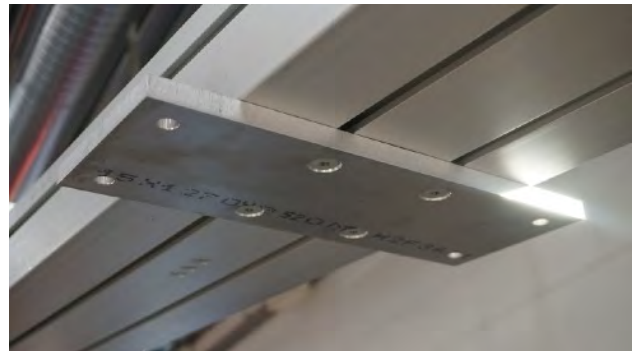
Remove the bracket / installation plate for transport
